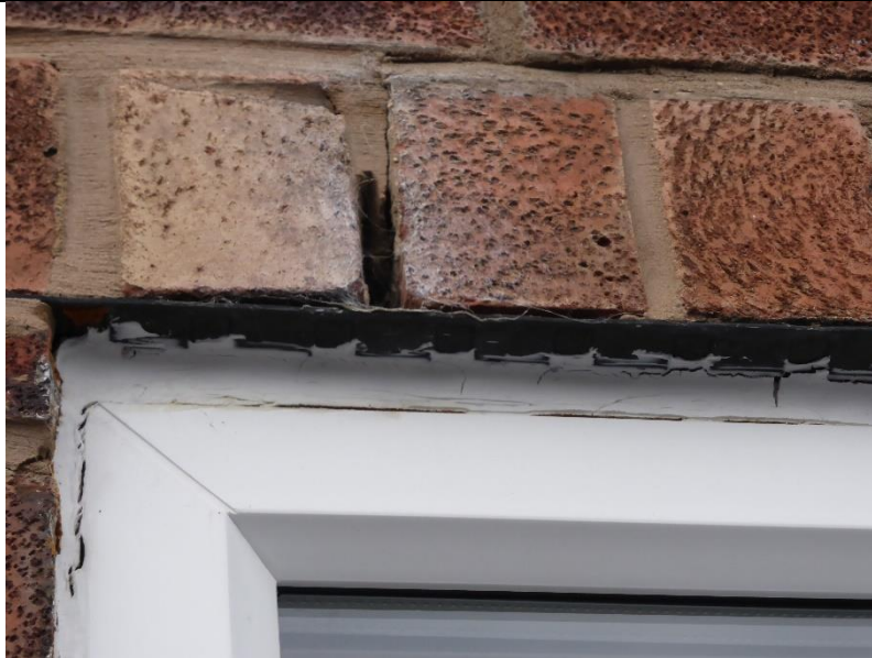
Plastic tray above the lounge window frame. A lintel is not visible
