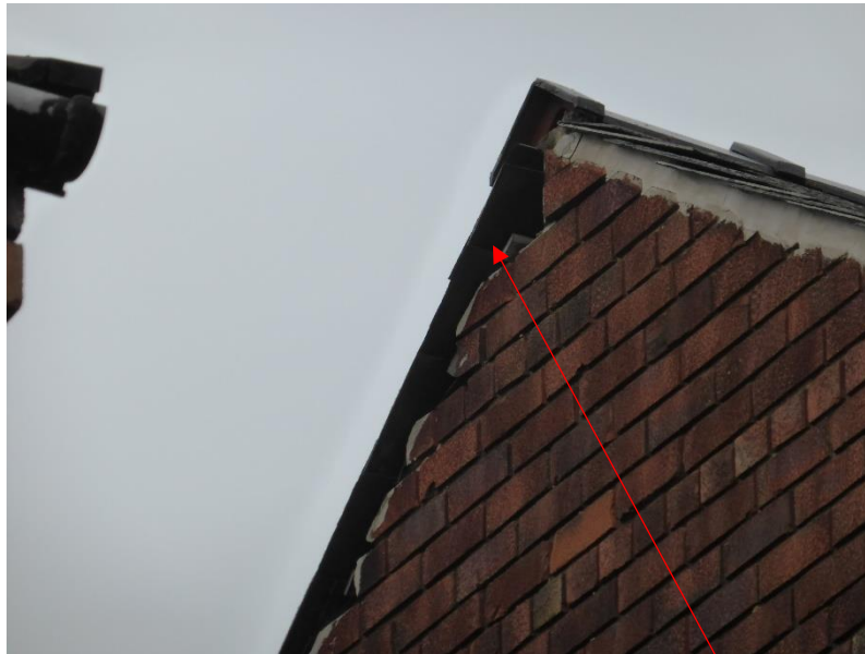
The underside of the roof is not sealed to the gable brickwork
