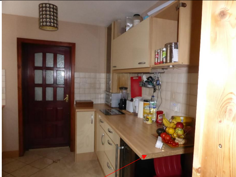
Note the edging is missing. Door and pelmet not fixed
