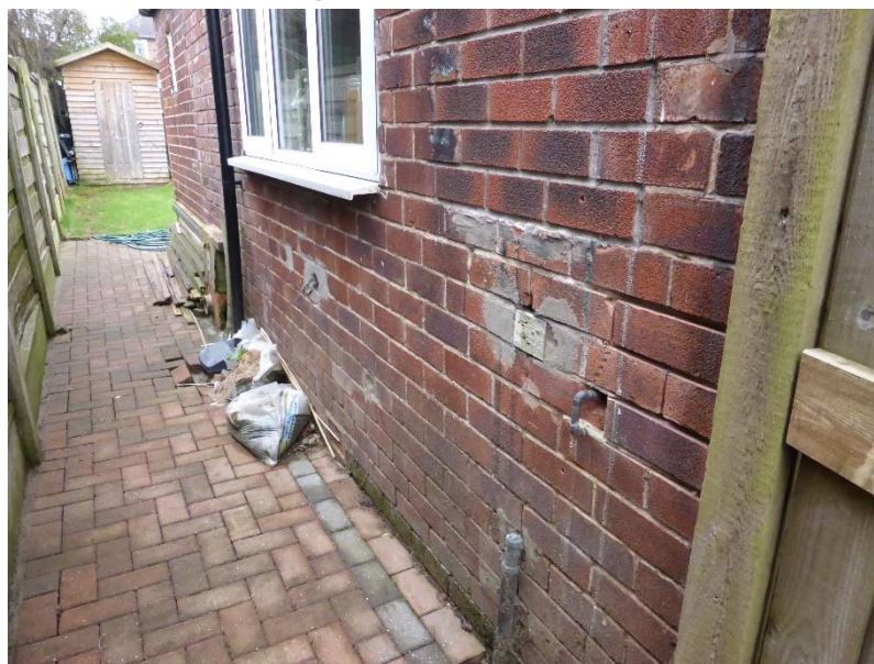
Block paving loose around the gully
