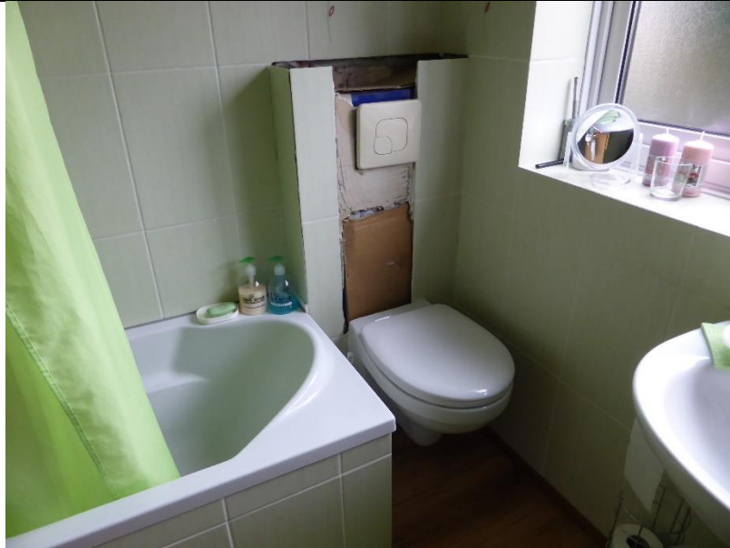
Tiles missing from back to wall toilet unit
