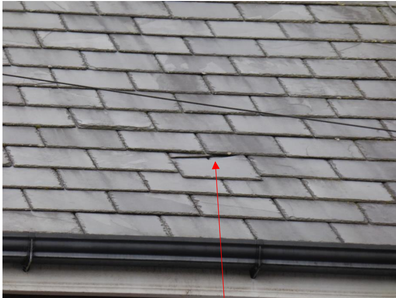
A cracked tile to the front elevation
