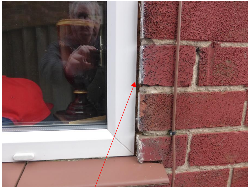
Sealant missing to the frame edge
