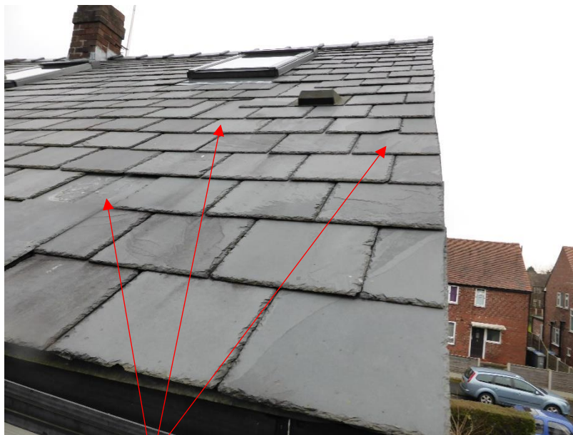
Some of the slipped and broken tiles to the rear elevation.
