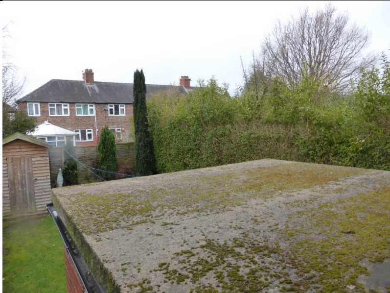
The concrete flat roof is covered with algae and is porous.
