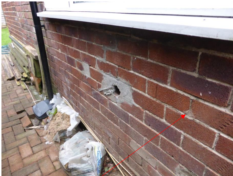
Evidence of injected insulation, note the untidy repairs and an open penetration
