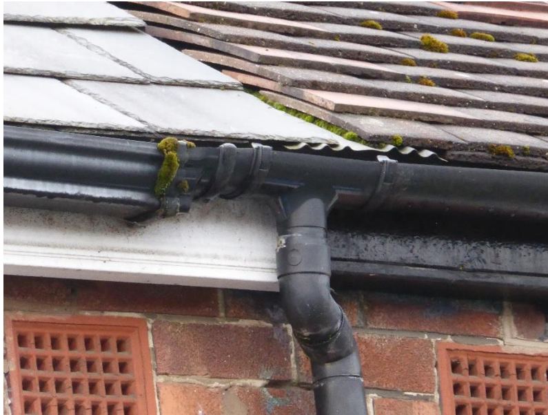
The two gutter types may be incompatible in this particular application
