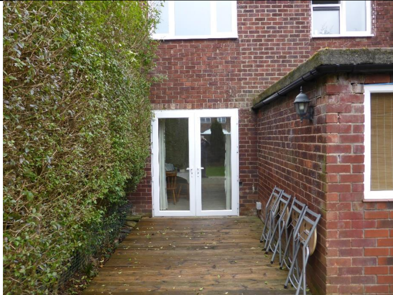
The decking planks sink when walked upon
