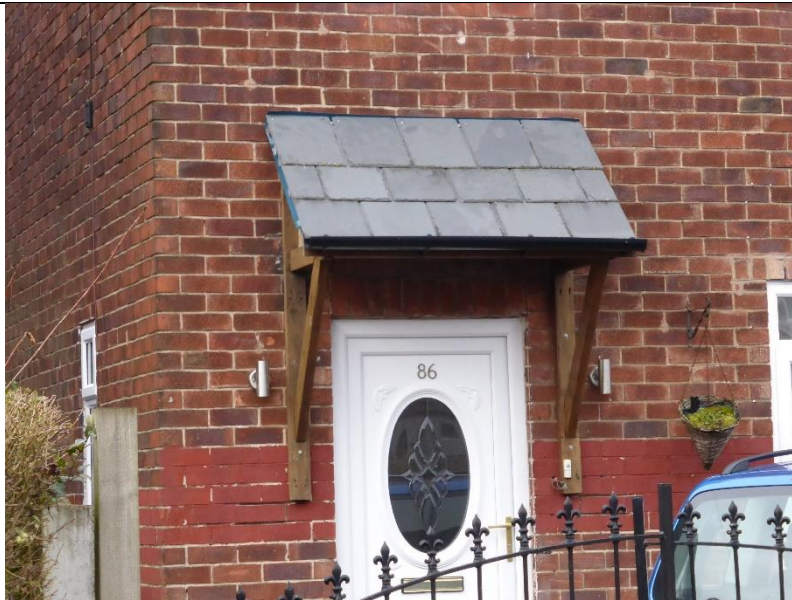
Lead flashing and pointing to the tile edges is required
