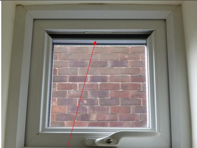
Landing window glazing bead missing
